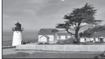
Point Montara Lighthouse
